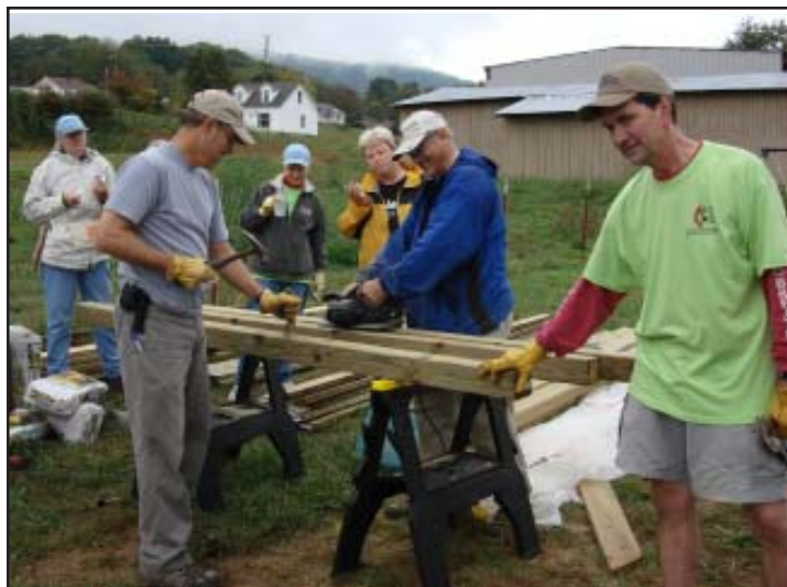
Last year's crew replaced crumbling front steps for a family
